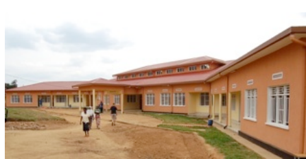
New Health Center in Gashora
